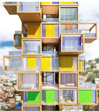
Tree House is the latest volumetric housing project developed by RSHP, to provide low-cost homes that can be rapidly assembled and deployed.
